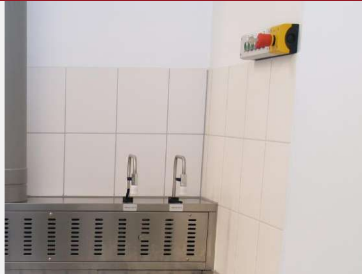
Top right: control system for dispensing unit with EMERGENCY-OFF button.
